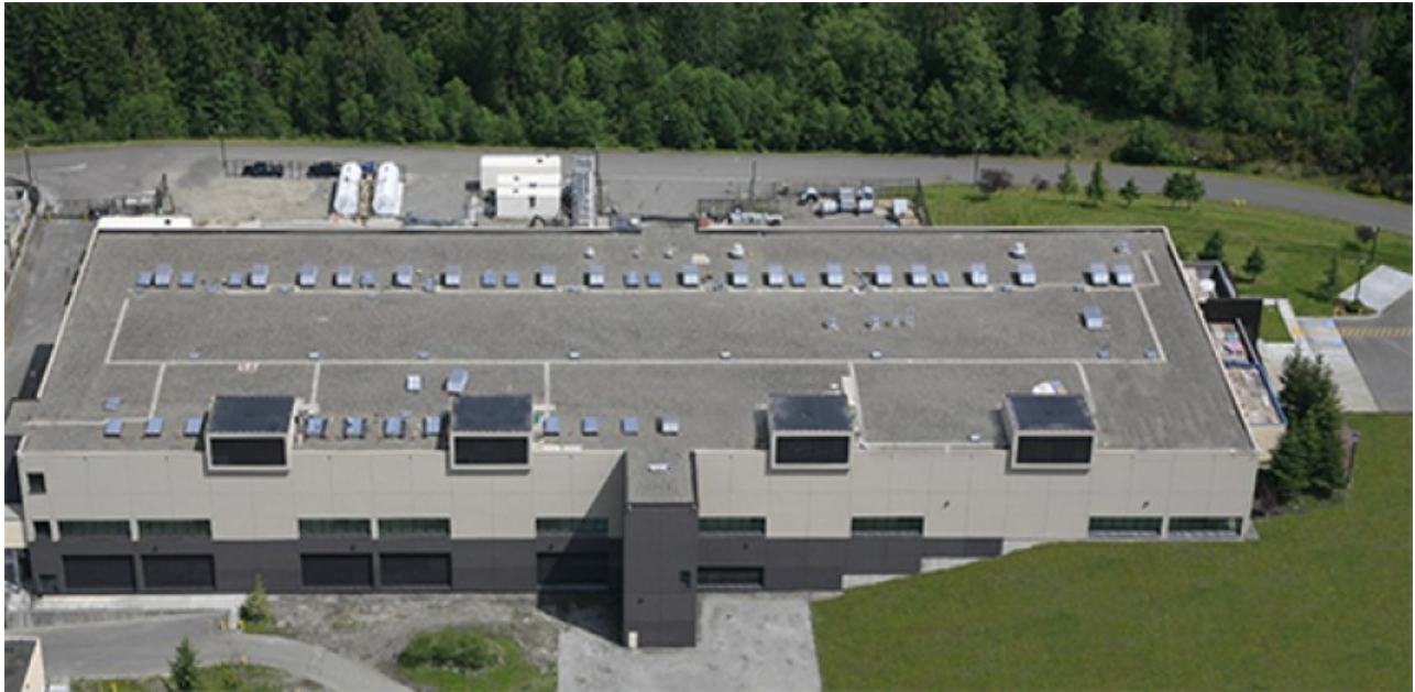
Centeris SH1 South Hill Data Center Seattle
